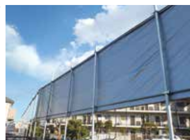
A chemical-proof shutter for preventing agricultural chemicals from scattering into the surrounding areas (Inagi City)
