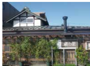
Facility prepared by reforming storehouse owned by garden owner
